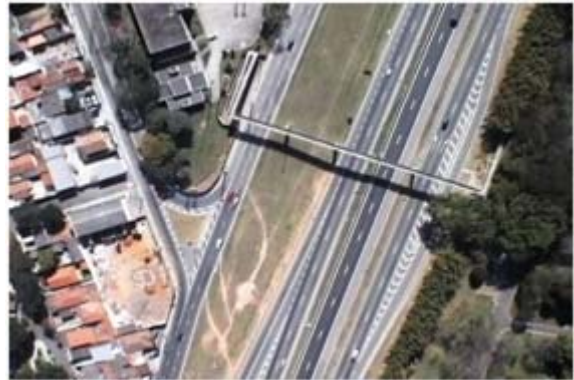
Figure 6 - Original Image Captured by the UAV.
