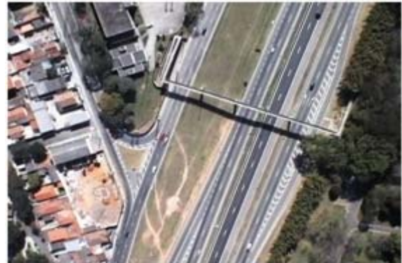
Figure 6 - Original Image Captured by the UAV.
