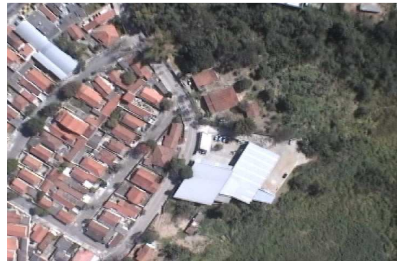
Figure 6 - Original Image Captured by the UAV.
